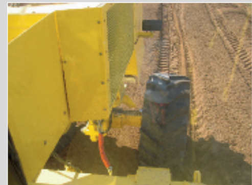
Excellent view over the working area and material field
