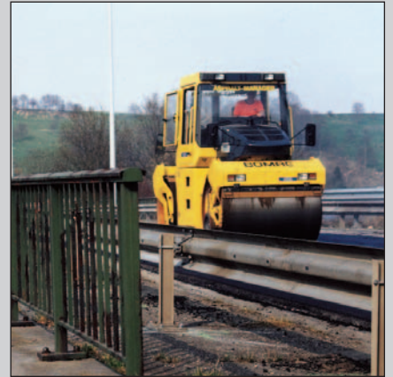
Compaction work on bridges or near housing requires low vibrations.
