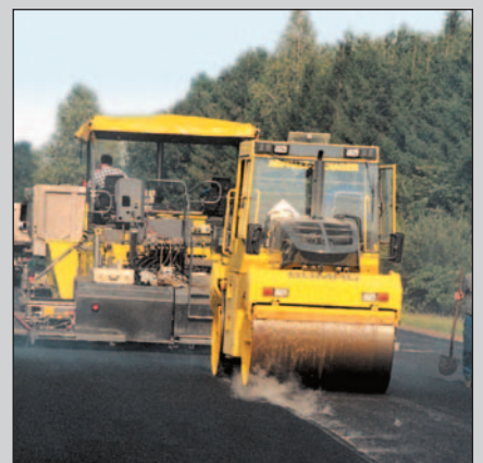
Compacting a longitudinal joint (hot on cold); amplitude is adjusted automatically.
