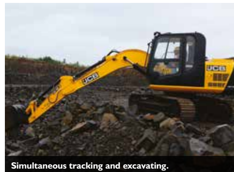
Simultaneous tracking and excavating.
