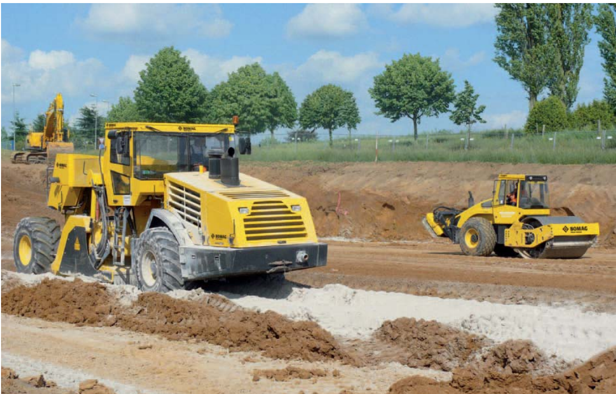
The BOMAG MPH 125 used as a stabilizer.
