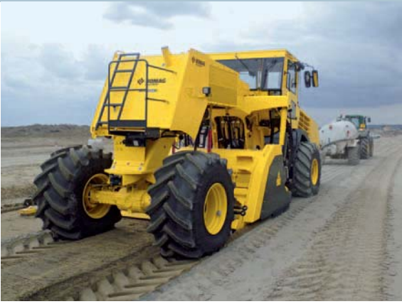
BOMAG MPH 125 on soil stabilisation ...
