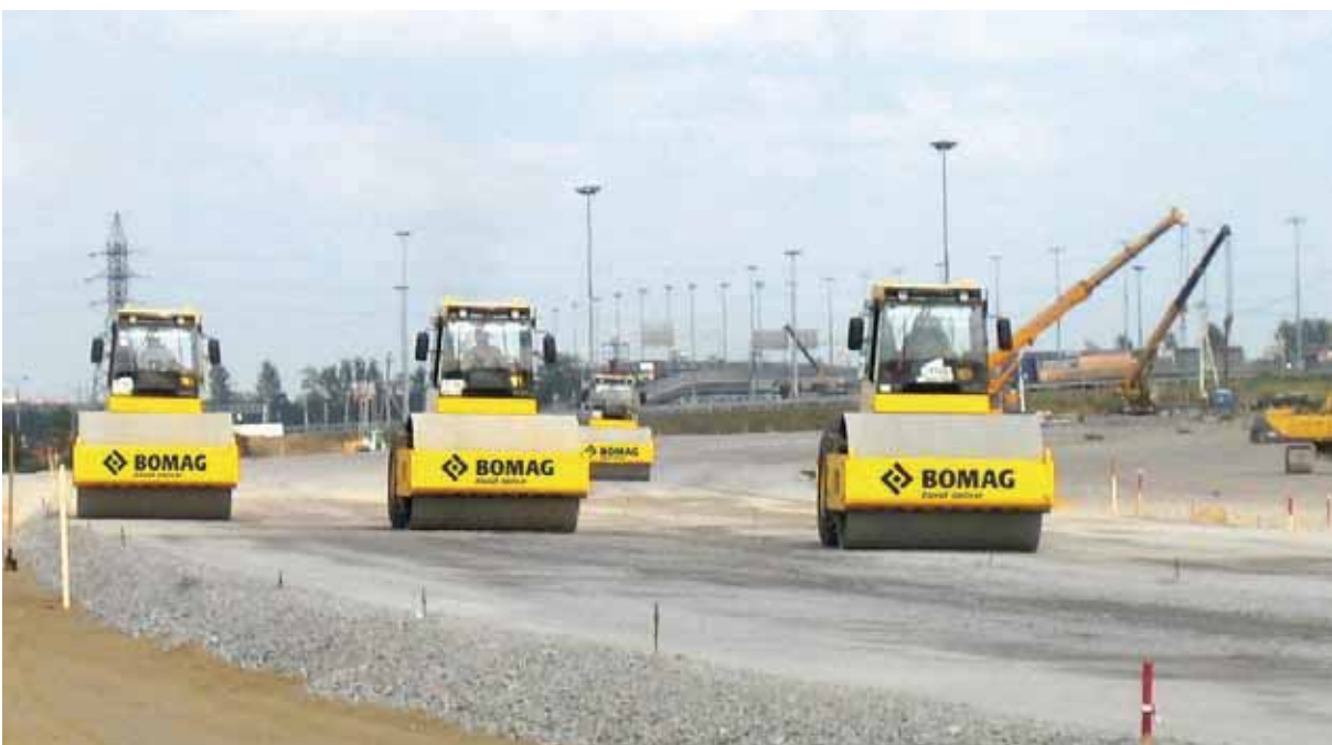
BOMAG single drum rollers on site in St. Petersburg.
